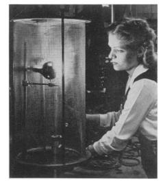
BRAZING by radiation is accomplished in the so-called hydrogen bottle shown in the picture. It is used in brazing copper parts by radiation from an incandescent filament which has a temperature of about 2,000 degrees Centigrade. The copper parts are heated to around 900 degrees.
