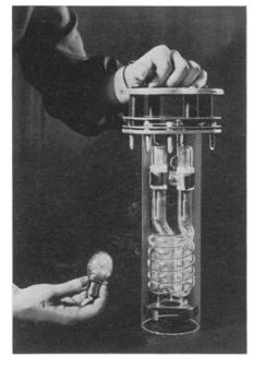
of lightning" from warplanes fitted with special electronic equipment. The tube, shown in picture beside a photo-flash bulb, permits taking countless night aerial photographs of any territory from altitudes up to two miles.
