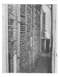
LOTS OF WIRE!—A behind the scene view of the complex wiring in the new electro-mechanical differential analyzer. The machine contains 200 miles of wire, 2,000 electronic tubes, several thousand relays, and about 150 motors.
