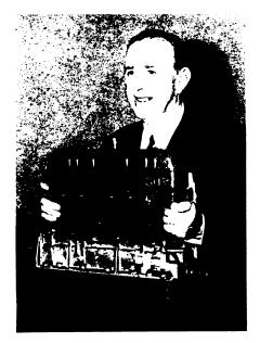
COMPACT ENGINE—The new 26-horsepower Crosley engine is built on a radically new principle from thin sheet-steel stampings and weighs only 59 pounds. Holding the engine easily on his lap is Powel Crosley, Jr., president of Crosley Motors, Inc.
