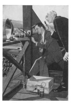
RADIO "HAMS"—The first invasion by amateur radio operators of a broadcast band used exclusively during the war by the Army and Navy for radar work was accomplished by W. C. White, right, electronics engineer of the General Electric Research Laboratory, and George H. Floyd, Electronics Department engineer. With the use of homemade equipment, they completed the first twoway radio telephone conversation on the 2300-3450 megacycle band between two buildings seven-tenths of a mile apart.
