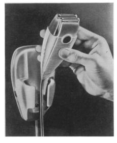
the razor is put in it. When the razor is taken from the holder, shown in the picture, the electric current is automatically turned on; when the shaver is returned, the current is cut off, and the cord disappears.
