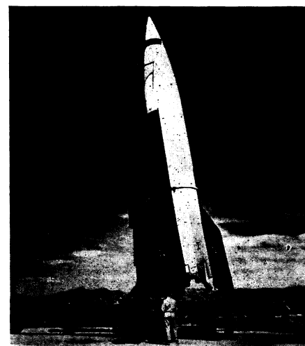
GAPA—This heretofore secret guided missile has been fired for the first time over the salt fields of Utah. It is pencil-slim, 10 feet long, and has been designed as potential defense against attack by enemy aircraft.
