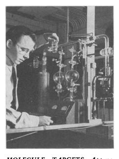
MOLECULE TARGETS—Apparatus reveals by microwave the kind of gas molecules present and the behavior of their atoms. The ammonia is contained in the glass bulb on the left. It passes into the long rectangular "barrel" or waveguide which extends across the lower part of the picture. When the vibrations of the gas are "in tune" with the vibrations of the microwaves, the microwaves are absorbed and a study of the absorption can be made. Research is being done at Westinghouse laboratories.
