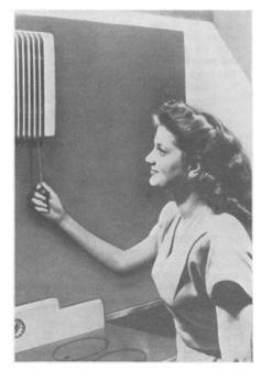
minimum resistance to air flow and is casily cleaned. The picture shows how it harmonizes with other installations. Its three-bladed propeller type fan is behind the grille.
