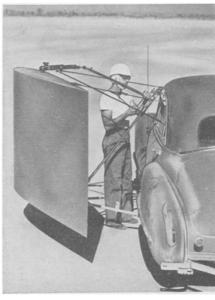
as shown in the picture, and offsets the centrifugal force of the vehicle racing around a circular track. With it, tire wear is about the same as on a straight highway.
