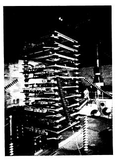
FOOD STERILIZING—The Capacitron, developed in the laboratories of the Electronized Chemicals Corporation, sterilizes and preserves food and drugs.
