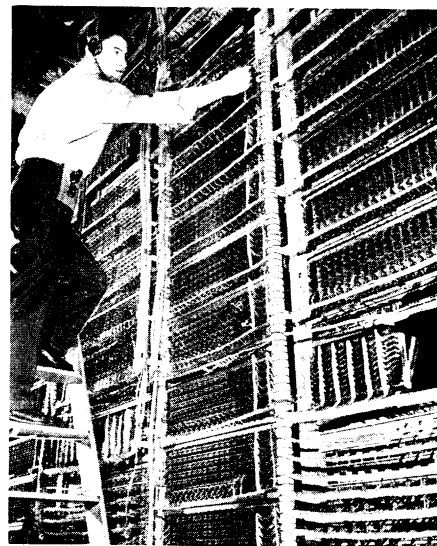
BELL'S BRAINCHILD —An important part of the telephone system, the main switching system at the Bell Telephone Laboratories duplicates every type of switching circuit in use in the telephone system today.
