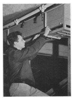
FIRE STOP—Gases and fumes from fires are sucked out through ducts, such as the one the operator is adjusting, by an exhaust fan. Sprinklers surround the ducts to cool the air and help block passage of smoke into the stair opening.
