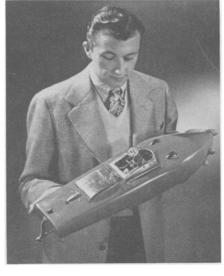
HYDROPLANE model, shown in the picture, is built from a kit around a plastic hull, all parts being jig-drilled to assure a perfect fit. It is powered by a tiny gasoline engine in an aluminum cowling. Pliers, screwdriver, file and countersink are the only tools needed to put the boat together.
