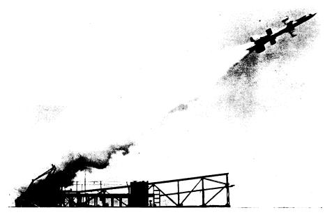
ENEMY AIRCRAFT INTERCEPTOR—This Convair Lark, officially designated XSAM-N-4, is a shipboard-launched guided missile designed to intercept and destroy enemy aircraft before ship or shore target can be attacked. The missile is powered by a high thrust, liquid fuel rocket motor and was built for the Navy's Bureau of Aeronautics by Consolidated Vultee Aircraft Corporation.
