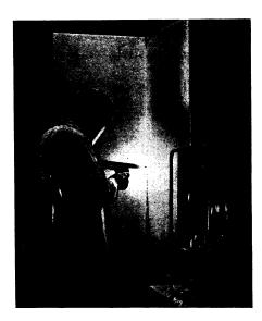
NEW WELDING GUN—Welding aluminum plate is made easy with this gun which has no rods to change, and the worker "lays his bead" without interruption. The filler metal is fed to the gun automatically from the spool at the right. This process will increase the use of aluminum plate in industrial fabrication.
