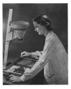
the picture, is a relatively efficient, economical type that uses a hollow sphere with a lamp burning inside. The white paint inside the sphere reflects and re-reflects the rays until the light is completely integrated, or evenly distributed.
