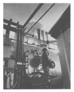
TEST CHAMBER—The center section of the test chamber shows the access door and some of the lead-ins for instrumentation lines. The two hoses attached to the door are part of a cooling system which jackets the entire chamber with a layer of water.
