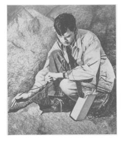
as uranium, thorium and radium. It contains a small Geiger tube, and the entire instrument is so constructed that it will operate even after being submerged in water.
