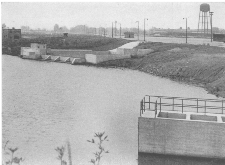
WATER CLEANED HERE —The "water laundry" cleans water utilized in industry so that it can be used again. It is known as a Gale Separator and, by baffles, separates sludge and grease from the dirty water
