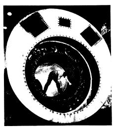
WHALE OF A GENERATOR— Largest generator equipped with Thermalastic insulation is this 100,000 kilowatt "whale" which seems to be in the act of swallowing the Jonah who is checking the Thermalastic-impregnated coils in the generator's stationary outer frame.
