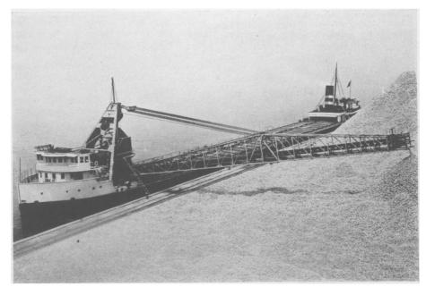
SELF-UNLOADING SHIP—Ten thousand tons of bulk cargo can be discharged and neatly piled ashore in about five hours, with as few as three men handling the conveyors and, if dock space permits, without assistance of any shore-based equipment. These ships, however, need not be built specifically for self-unloading. Successful conversions have been made of cargo ships that have operated for as long as 30 years by old-fashioned methods of unloading.
