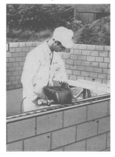
blocks without the skill required in trowel application and with less waste. It is an electrically-operated device with an endless screw inside of the type used in familiar meat grinders.
