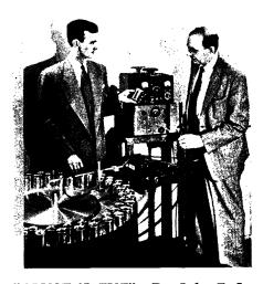
"CRYSTAL EYE"—Dr. John E. Jacobs, GE X-Ray Corp. research engineer (left), is holding a partly filled can of baby food which has been spotted by a new testing apparatus. Heart of the apparatus is the little crystal holder facing the cans from the left. Dr. Jacobs and Dr. Rudolf Frerichs, physicist of Northwestern University (right), developed the crystal.
