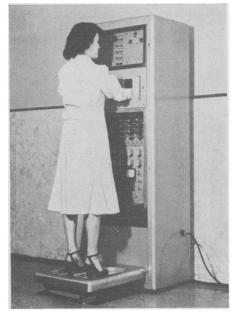
S RADIATION detector, for personnel using radioactive materials, checks hands and feet at the same time. The person stands on the device, as shown in the picture, with hands in checker pockets and feet on a checker platform. A beta-gamma count registers automatically in five seconds.
