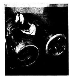
JET ENGINES—Although these two jet engines have equivalent diameters, the new Allison J35-A-23 on the left is much more powerful than its predecessor, yet fuel consumption has been cut considerably. Looking over the engine are Henry Devaney, engineer, and Frank Herdrich, foreman.
