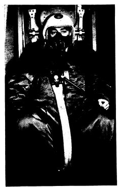
QUICK EJECTION—Easier escape from the seat of their planes for jet pilots comes from combining the four leads, wires that connect a pilot to his plane and its equipment, into one long rubber cable that can be separated from the plane when the ejection seat is lever triggered.
