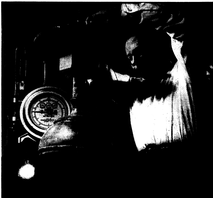
SUPER VACUUM BOTTLE —Keeping the world's coldest liquid is the job of this new vacuum bottle designed by Dr. Aaron Wexler of Westinghouse Research Laboratories. He is lifting the "bottle" from a bath of liquid nitrogen.
