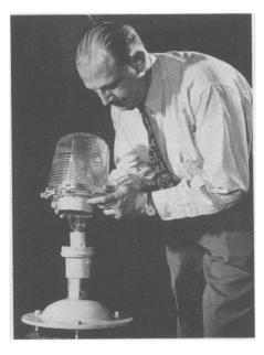
as shown in the photograph. Two flattened sides of the lens emit high candlepower beams along the runway, a curved side
