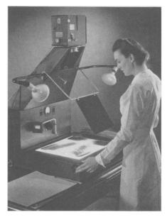
copies on a single roll of film. To use, the radiograph is placed on an illuminator surface and a button pushed.
