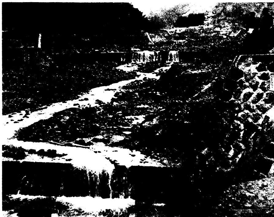
"SABO" WORKS —Shown here is one of the main weapons—check dams in stream channels—used by the Japanese in fighting the battle of stream erosion. Revegetation of the eroded slopes is a related activity. Designs and results of Sabo Works need thorough investigation.
