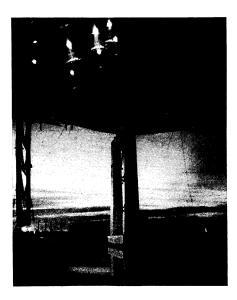
PASSAIC RIVER BRIDGE—to take advantage of high tide and low winds, two of the giant 173-ton haunch girders used to make the Passaic River Bridge were erected at night. This picture shows where the work to complete the longest girder span bridge
