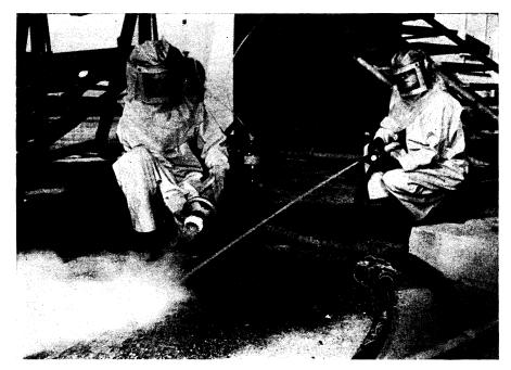
ROCKET FUELER—To save time in fueling rockets, Republic Aviation Corporation developed the first mobile rocket engine servicing truck that carries the two propellants and pressurizing gas required for rocket propulsion. Here one of the liquid oxygen lines is being "bled" before being attached to the engine tank, while the ground is sprayed with water to reduce fire danger.
