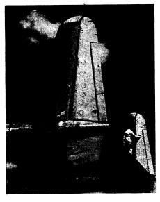
FLYING BOXCAR IMPROVED— The new ventral fin that has been added to the U. S. Navy's R-4Q is shown in the close-up photograph. The plane is designed as a tactical and strategic military cargo aircraft for use under combat conditions.
