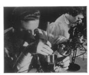
ASSEMBLY PROBLEMS, such as fixing hair-thin wires to barely visible germanium wafers, are solved by new tools and mechanized techniques. Finished transistors withstand great vibration and shock. Engineers see many opportunities for these rugged devices in national defense.
