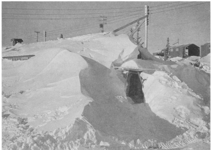
SNOWBOUND IN THE ARCTIC —This snow-covered but illustrates one of the problems encountered in Arctic life. Drifts often bog equipment and endanger personnel. Winds shift snow into the streets if buildings are not situated properly relative to the wind. Even the drifts created by snow plows are dangerous.
