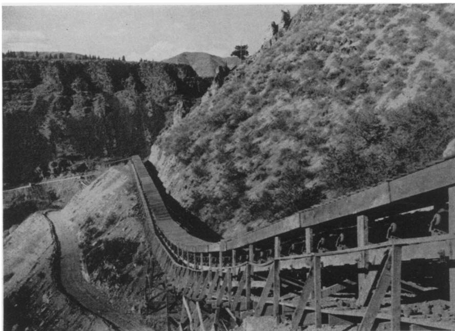
TRANSPORTING CLAY —This conveyor belt, used to carry clay two miles from the pit to the Anderson Dam in Idaho, was installed with a cover to protect the clay en route from sun and rain.
