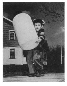
CARBOY BOTTLES for shipping poisonous or corrosive chemicals safely are blow-molded of a light-weight, polyethylene plastic as shown in the photograph. The containers are so rugged that the steel treads of a 10-ton bulldozer failed to damage
