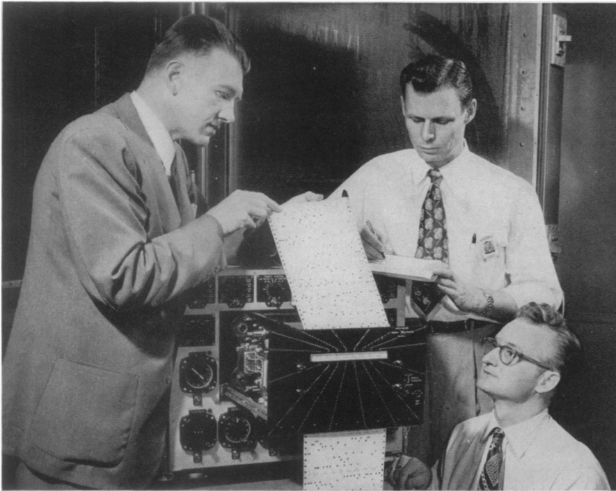
PUNCHED TAPE CONTROLS —A complete flight can be flown with such a punched tape giving orders to a robot autopilot designed by Minneapolis-Honeywell engineers.
