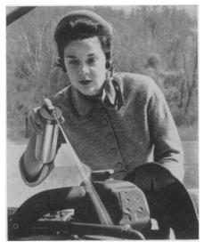
show, has a one-pint capacity and puts out most gasoline, oil and grease fires as well as those due to defective electrical equipment. Using carbon tetrachloride as the basic fire-fighting ingredient, the compact extinguisher shoots a 25-foot stream. It is shown in the photograph.
