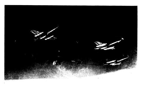
THREE AT A TIME—Multiple refueling of three Meteor jet fighters at the same time has been accomplished by a U.S. Air Force B-29, using the probe and drogue system manufactured by Flight Refuelling Ltd., Dorset, England.
