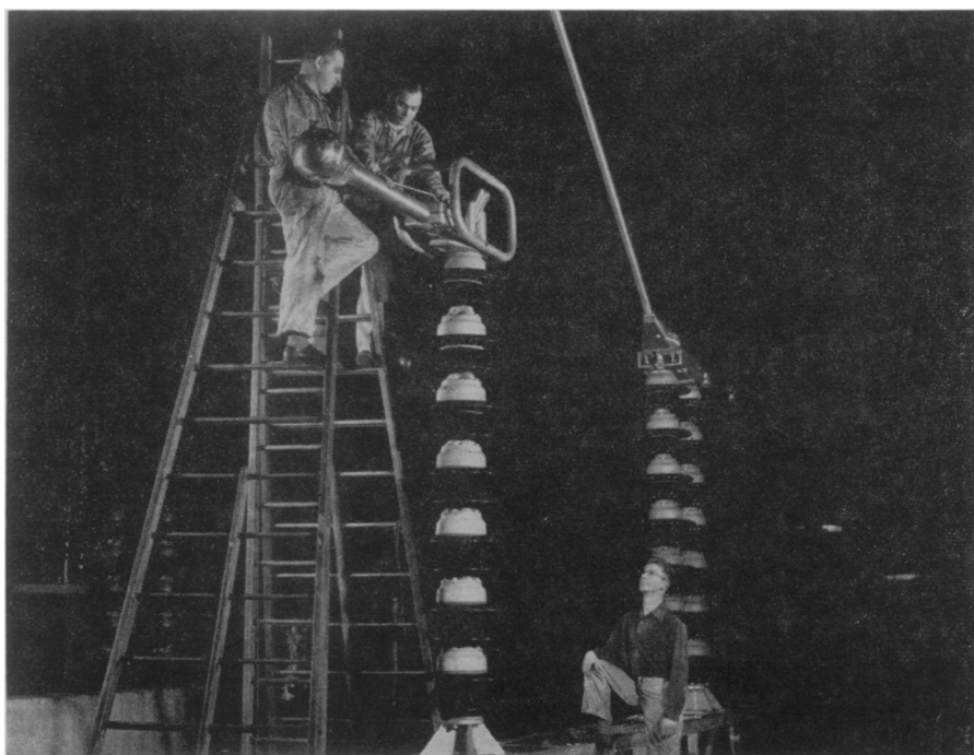
SUPER-SWITCH —This giant switch for electric utilities can withstand a lightning stroke of 1,300,000 volts. The switch blade, about 17-feet long, can be operated manually or by an electric motor.
