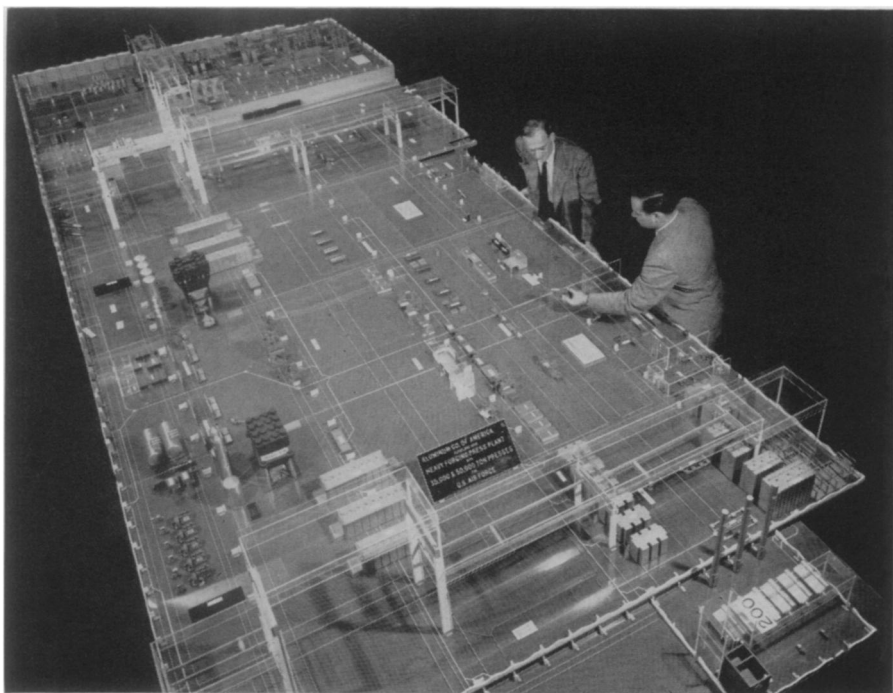
MODEL PLANT —The scale model of the Air Force heavy forging press plant being built at Alcoa's Cleveland works. Use of the layout allowed shop foremen to contribute their knowledge to the final plans.
