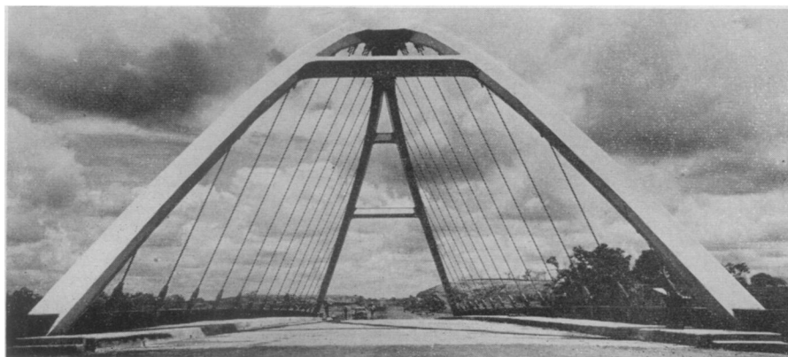
STEEL BRIDGE SPAN —Freedom of form previously available only with concrete has been achieved with steel in the bridge spanning the Río Blanco River near Vera-Cruz, Mexico, shown here. The structure was designed by Dr. Thomas C. Kavanagh of New York University. Camilo Piccone of Mexico was the engineer of this span, which has slender arch ribs free of cumbersome bracing.
