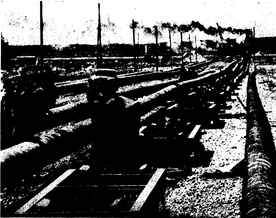
LABOR-SAVING DOLLIES —Rushing to complete the laying of two four-mile sections of 20-inch pipe along the bottom of Mackinac Strait before the winter freeze, contractors saved more than 100 miles of land clearing and ditching by crossing the 240-foot deep shipping channel with this submarine pipeline. The tires were used on pipe-launching devices that put pipe in the water at the rate of almost 1,000 feet per hour.
