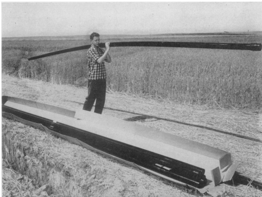
PLASTIC PIPE —Used in a pipeline more than nine miles long near Poplar, Mont., one length of plastic pipe, held here by 14-year-old Richard Thomas, weighs only 13 pounds as compared to a comparable length of steel pipe, which would weigh 153 pounds.
