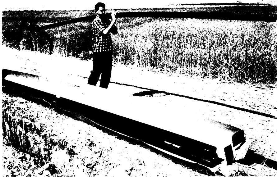
PLASTIC PIPE —Used in a pipeline more than nine miles long near Poplar, Mont., one length of plastic pipe, held here by 14-year-old Richard Thomas, weighs only 13 pounds as compared to a comparable length of steel pipe, which would weigh 153 pounds.
