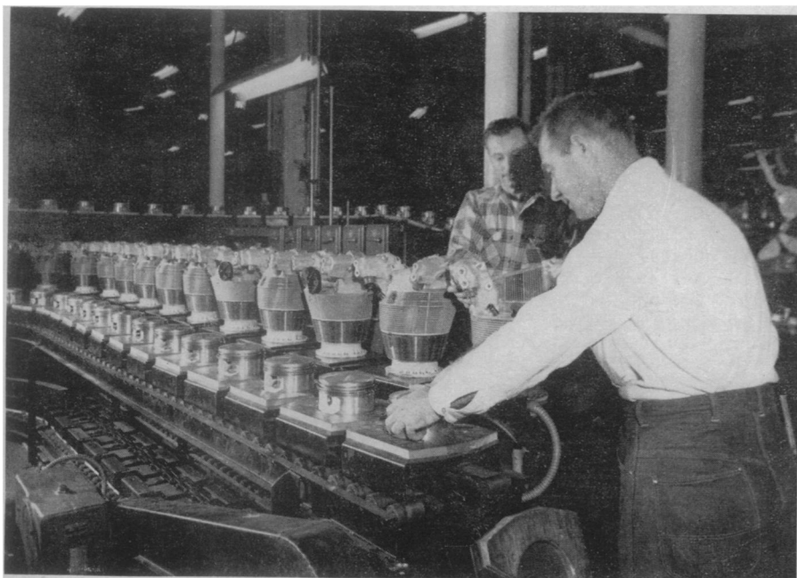
ASSEMBLY-LINE TURBO ENGINES —Factory conveyor line carries assembled cylinders and pistons to operators in order to speed-up installation on the engine at the restyled Curtiss-Wright plant, Wood-Ridge, N. J.
