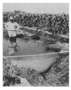
M PLASTIC IRRIGATION dams can be folded up and carried about due to their light weight. Stretched across an irrigation ditch and over its banks, the dam is held in place by the weight of water it retains, as shown in the photograph. Made
