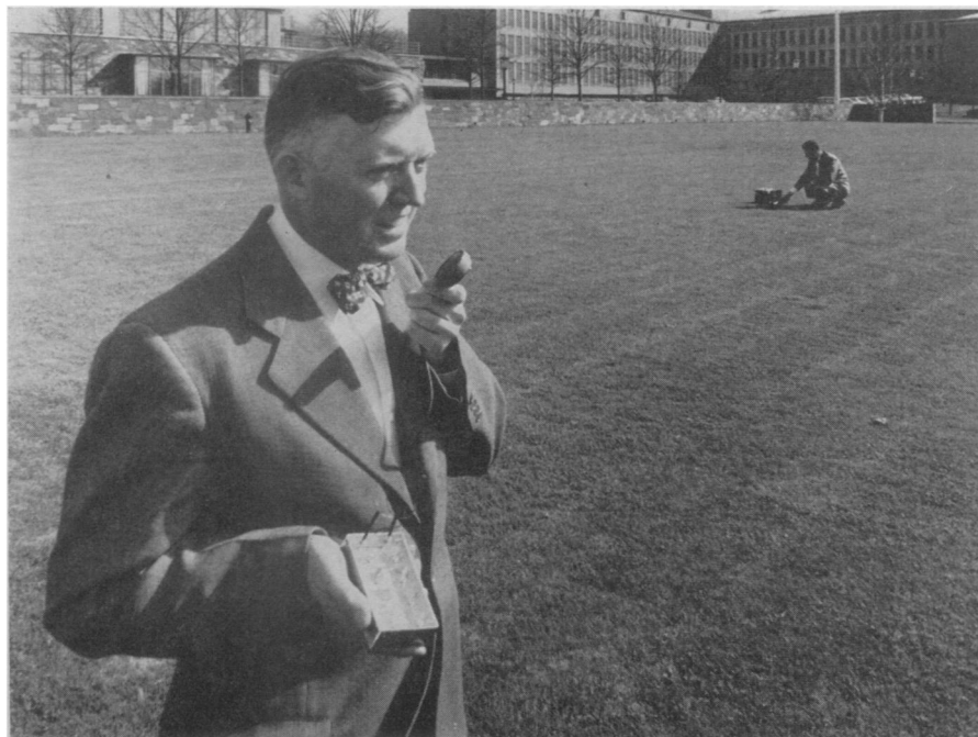
SOLAR POWER SOURCE —The sun's rays falling on the solar battery are the only source of power needed to operate a small mobile radio transmitter. Here D. E. Thomas talks to M. B. Prince across the lawn at Bell Telephone Laboratories.
